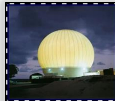
Ground Based Radar - Kwajalein (GBR-K) Capability Phased Array – X-Band
