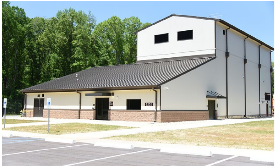
The Directed Energy Systems Integration Lab is a 5,400-square-foot facility designed to provide the Army with a consolidated capability to support a full end-to-end directed energy system, from software simulation, to subcomponent system testing, subsystem testing and full system verification and validation testing. The lab, dedicated Aug. 8, 2022, is located on Redstone Arsenal, Alabama. (U.S. Army photo by Carrie David Campbell)
