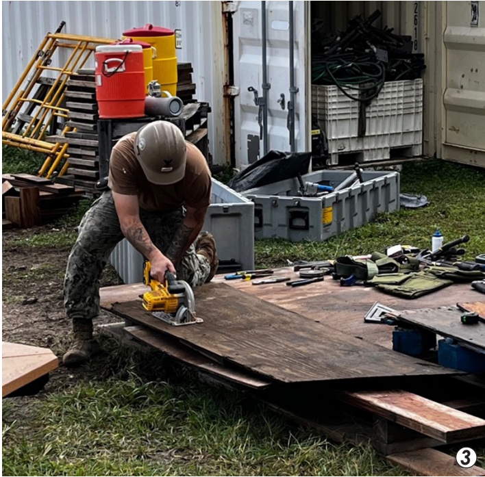
AG-KA Commander Col. Tom Pugsley for her role as Project Safety of the Richardson Theater on May 23 during an awards ceremony. 3) Equipment Operator Second Class Ricardo Najera cuts plywood for use in prepping for a sidewalk placement on May 27.
