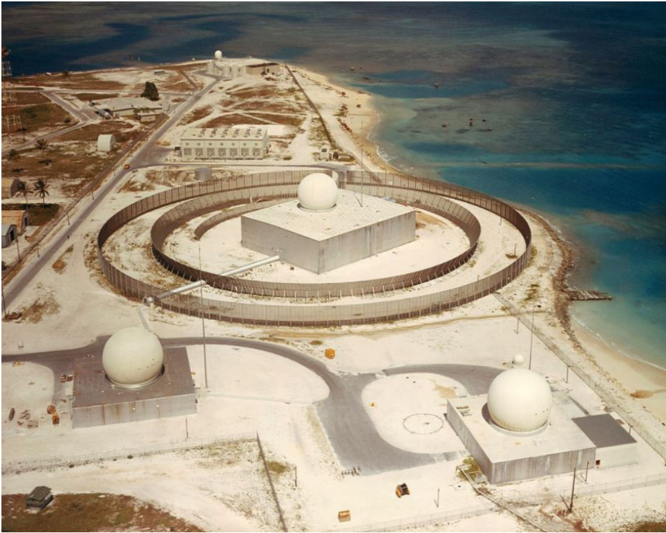
In this July 20, 1963 U.S. Army Space and Missile Defense Command photo, the raised radome of the Zeus Discrimination Radar is visible in the center of reflective rings of clutter fencing. The metal tunnel running between the ZDR building and the outermost fencing provided protected access to the radar during operations. Missile-tracking radars are visible in the far-distant background.
