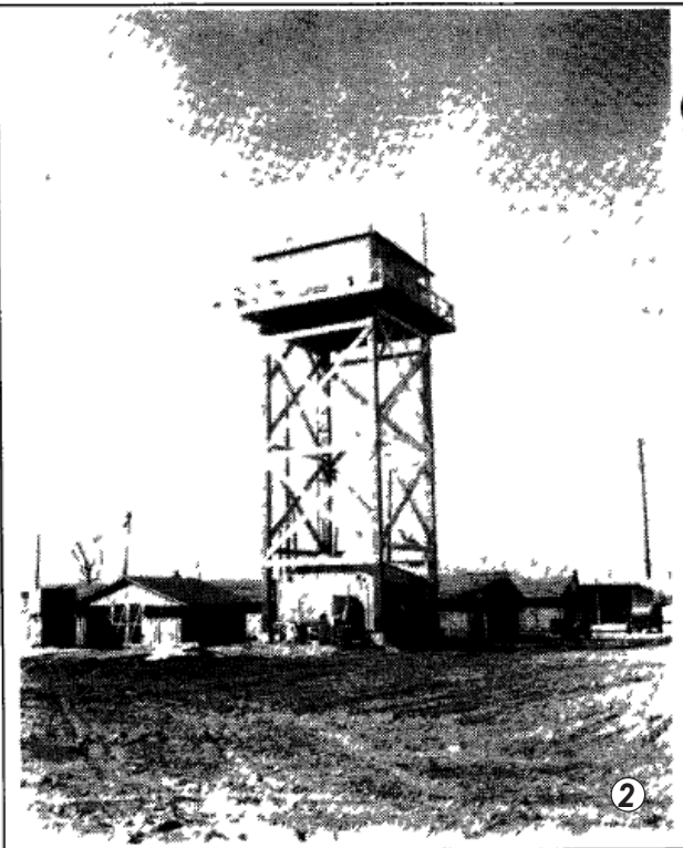
(1) This temporary control tower, constructed of coconut palm logs, was used to direct planes on Kwajalein (photo taken Feb. 9, 1944). (2) A permanent control tower stood completed March 26, 1944. This tower was first erected too close to the taxiway and was moved back 25 feet, intact.
