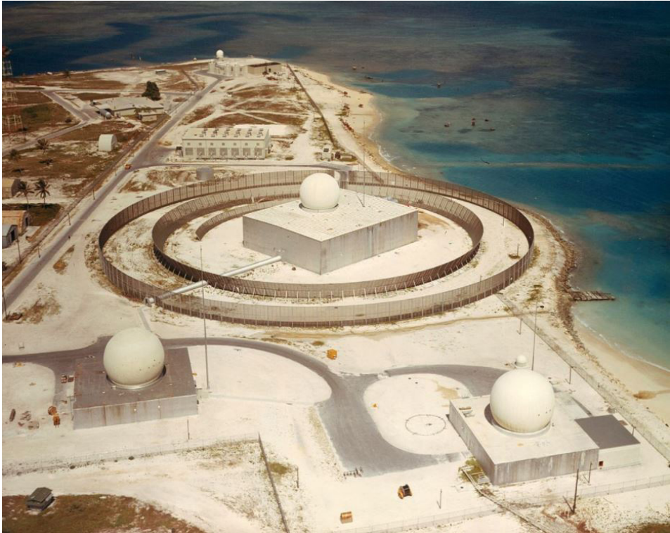
In this July 20, 1963 USASMDC photo, the raised radome of the Zeus Discrimination Radar is visible in the center of reflective rings of clutter fencing. The metal tunnel running between the ZDR building and the outermost fencing provided protected access to the radar during operations. Missile-tracking radars are visible in the far-distant background.
