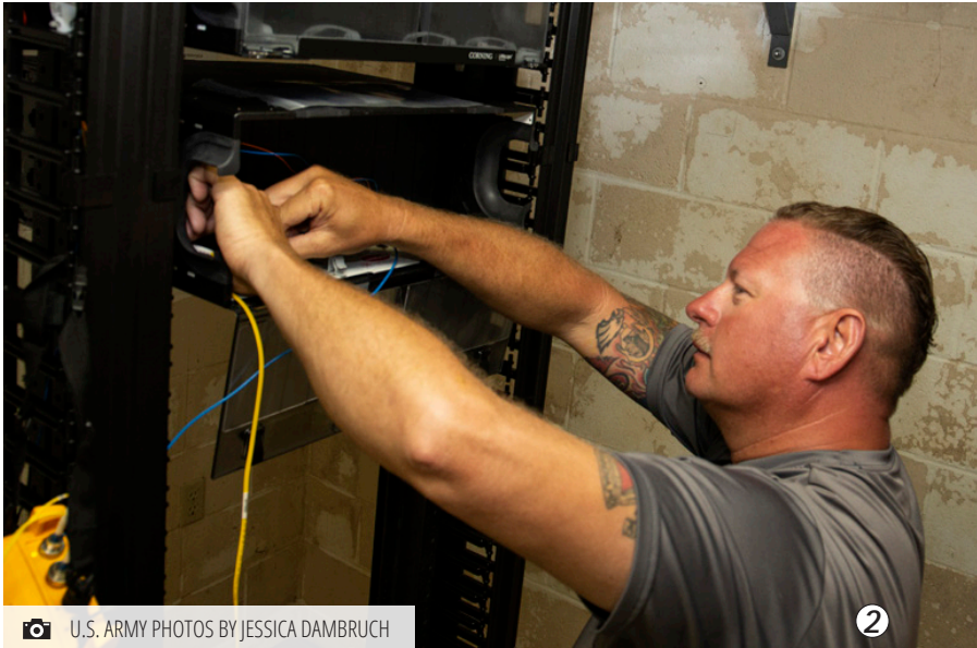
1) Alfonse Zito assists with testing George Seitz Elementary School's new voice and data infrastructure in the main classroom hallway . 2) Jamie Johnson checks out the wiring at a neighborhood network cabinet near George Seitz Elementary School. The system is designed to support upgrades in the years to come.
