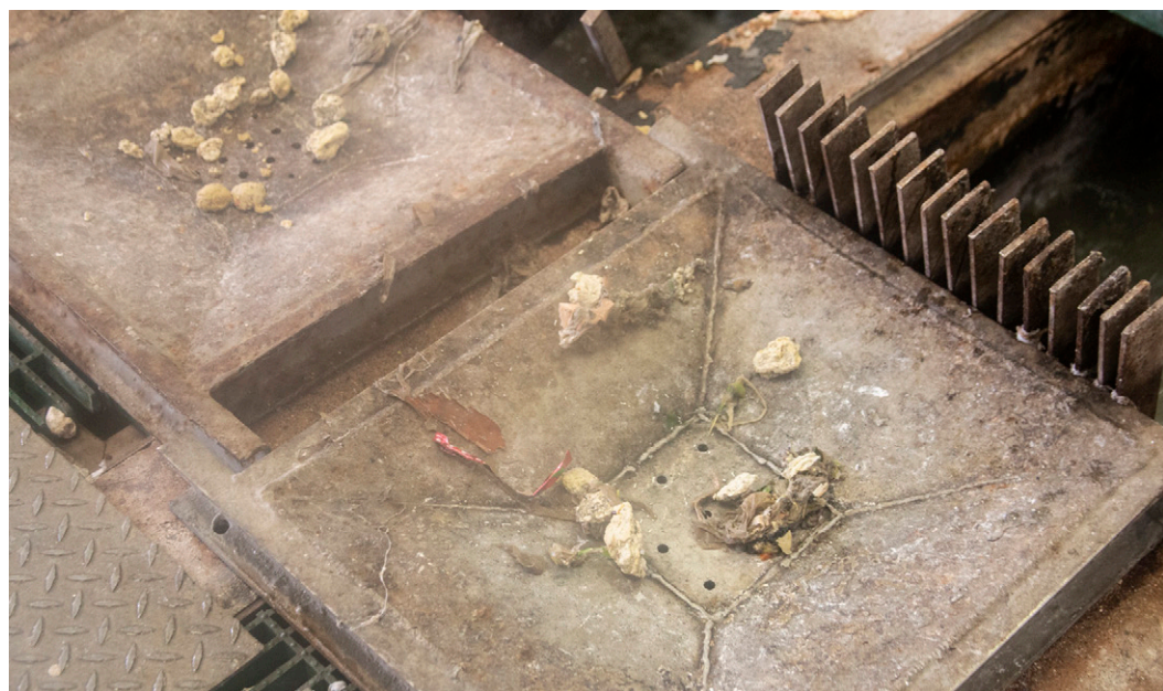
Pictured here, congealed grease is removed from the wastewater supply early in the treatment process.
