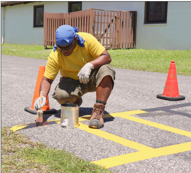
KRS construction crew member Bildon Joran applies the finishing touches to a crosswalk behind George Seitz Elementary School, August 8.
