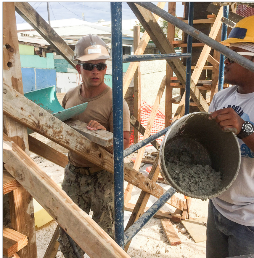
LEFT: Builder Constructionman Alex Kifolo, from Lancaster, Pennsylvania, cuts lumber during an NMCB-1 school construction project on Ebeye. RIGHT: Builder Third Class William Mathis, from Southampton, Virginia, and local apprentice Junior Jibke place concrete into column formwork during the build.
