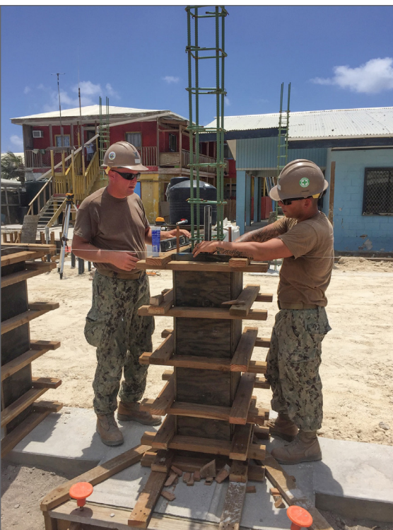
Builder 1st Class Jesse Koehn, from West Bend, Wisconsin, and Builder 3rd Class William Mathis, from Southampton, Virginia, set column form-work during a project at the Ebeye school.
