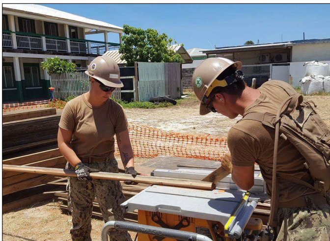
Builder Constructionman Emma McCarthy and Builder Constructionman Alex Kifolo prepare lumber for concrete formwork on a schoolhouse construction project with apprentice Junior Jibke, March 31.
