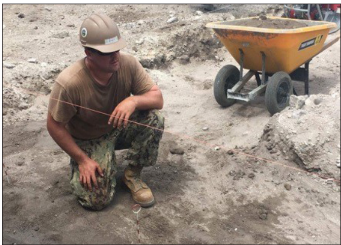
Utilitiesman 3rd Class Jeffrey Baer of Naval Mobile Construction Battalion 1 checks the locations of column footers for a school building project, April 22.
