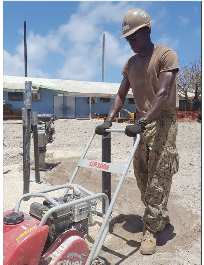
Construction Electrician 2nd Class Junior Jeanbaptiste uses a vibrating sled to compact the dirt throughout the Ebeye school building project construction site, May 1.
