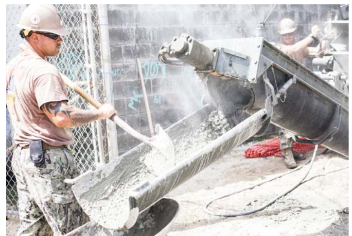
A crewmember pushes newly-mixed concrete down a chute from the team's mobile mixer into wheelbarrows for the Seabees.
