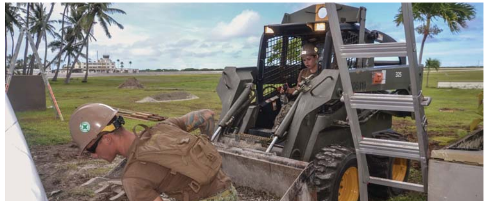
Equipment Operator 3rd Class Nathan Suhy and Equipment Operator Construction Apprentice Bridget Osborn transport and spread gravel along the base of the Vet's Hall to improve stormwater drainage away from the building.
