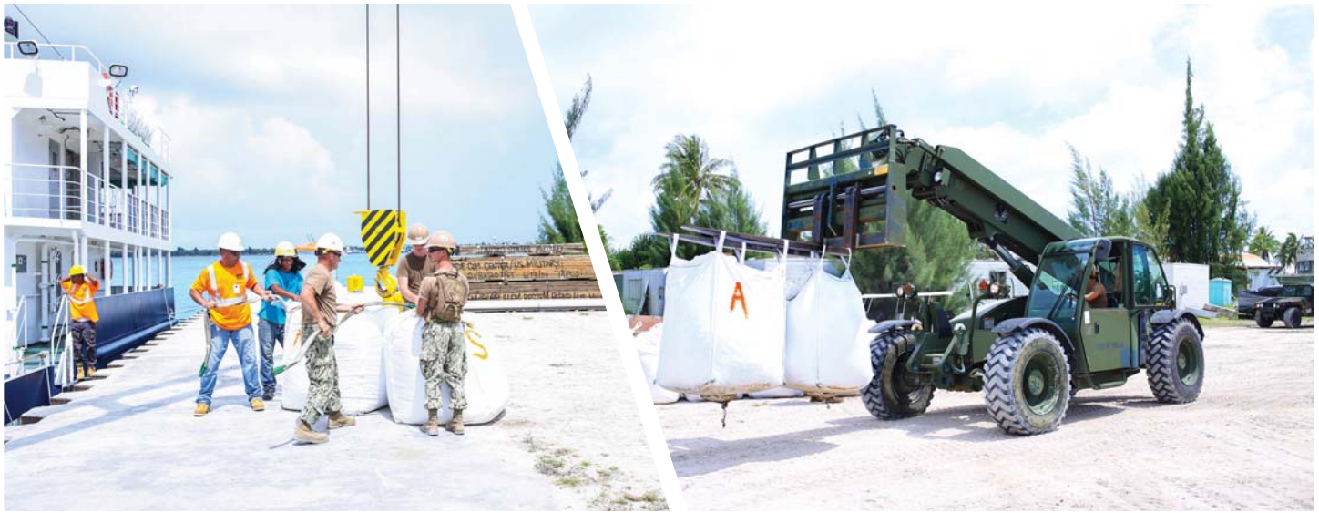
LEFT: Seabees working with Construction Civic Action Detail-Marshall Islands help prepare 1.5-ton bags of concrete aggregate for transport. RIGHT: A Seabee hauls off some of the 375,000 pounds of aggregate needed for development builds on Enniburr and Ebeye.
