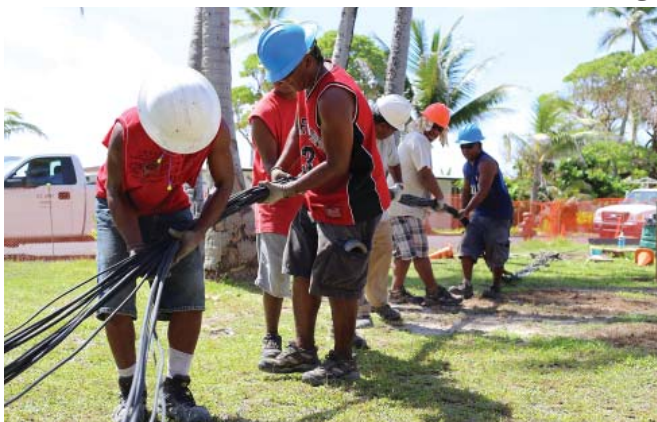
An Electric Shop crew helps feed a set of heavy electrical lines underground to the location of the distribution vault.
