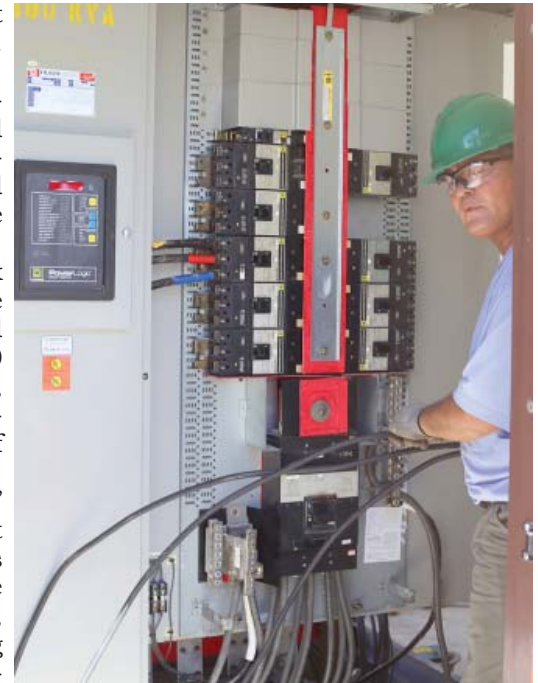
Kobok Aron, a journeyman electrician with the Electric Shop, attaches housing wiring to a set of circuit breakers on the transformer at the intersection of Ocean Road and Fifth Street June 28.
