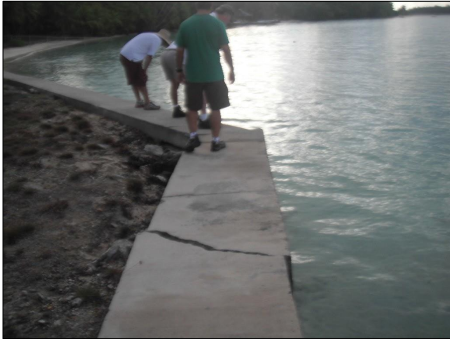
Figure 2 – Cracking was evident on the abutment near the Yokohama Pier area.
