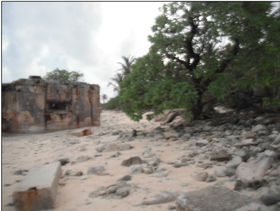
Figure 3 – Inadequate riprap was observed near the pillbox area.
