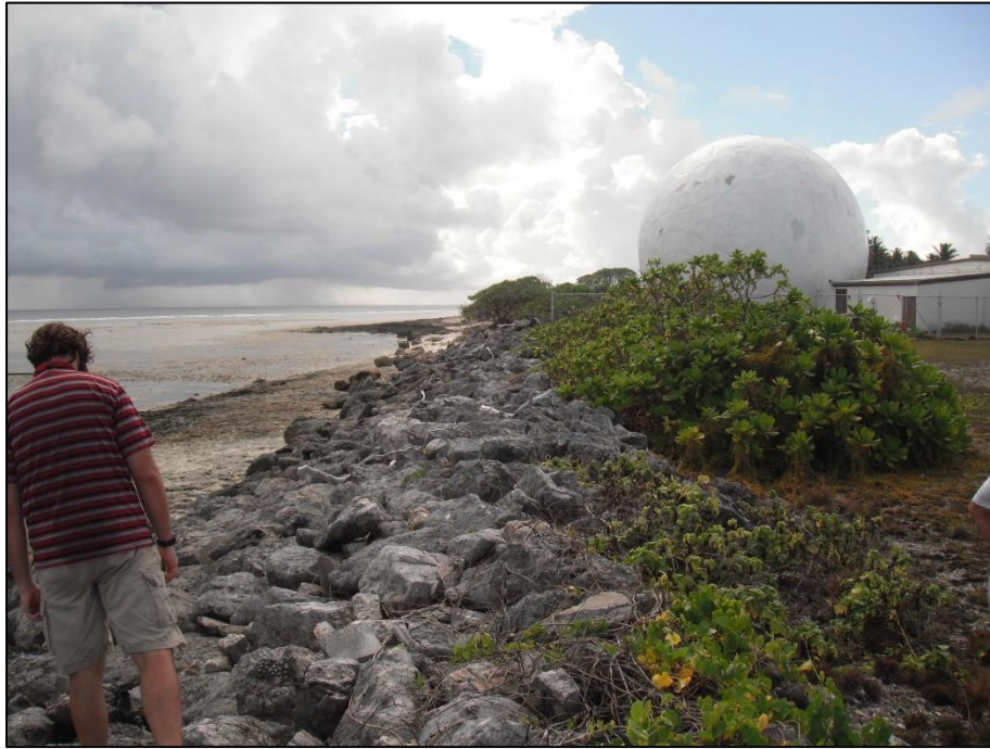
Figure 11 – Insufficient shoreline protection allows seawater breaching.
