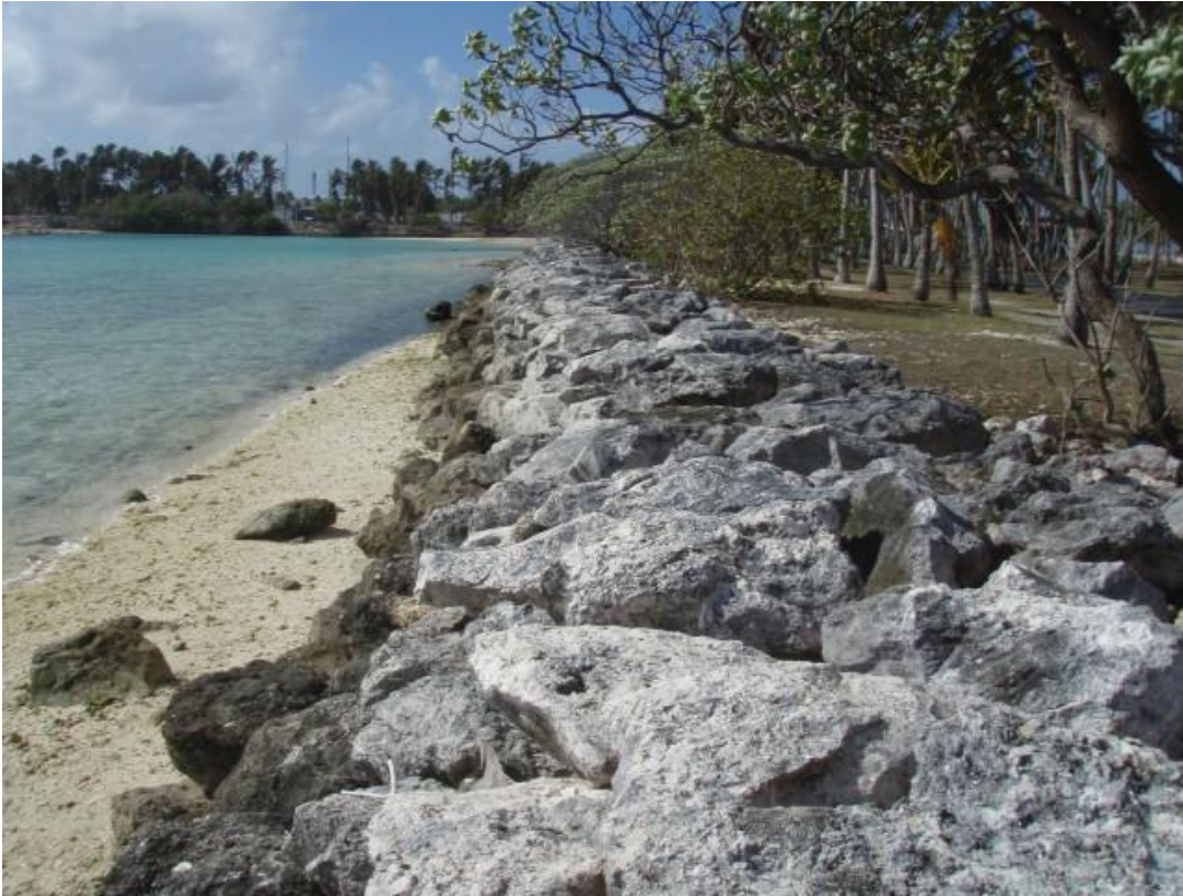
Figure A4: Revetment with rock armor stones located on Roi-Namur.
