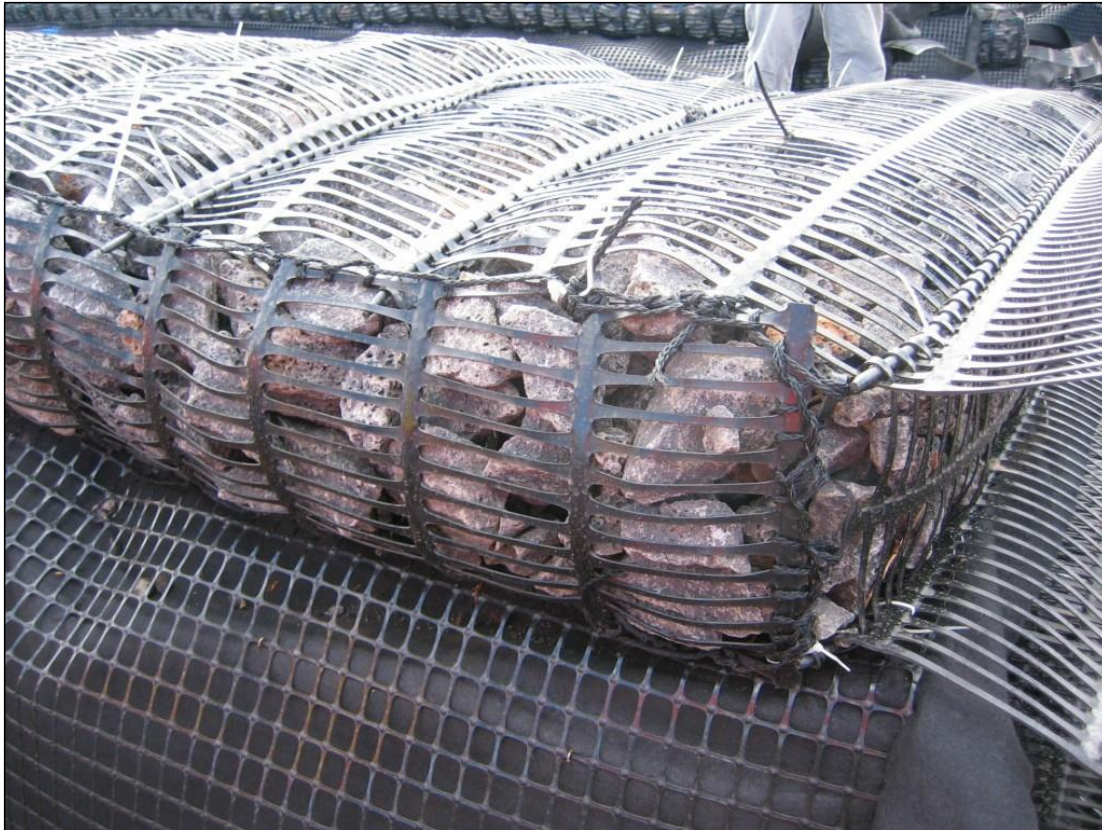
Figure A1: Rock filled marine mattress with underpinned geotextile fabric.
