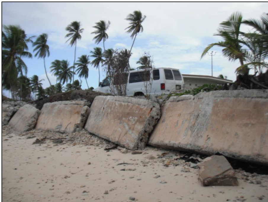
Figure 5 – Concrete slabs previously placed as emergency shoreline protection.
