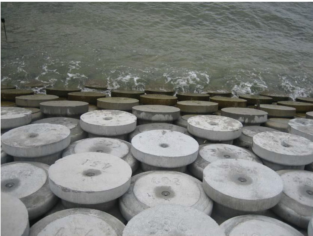
Figure A5: Samoa Stone concrete armor unit revetment.
