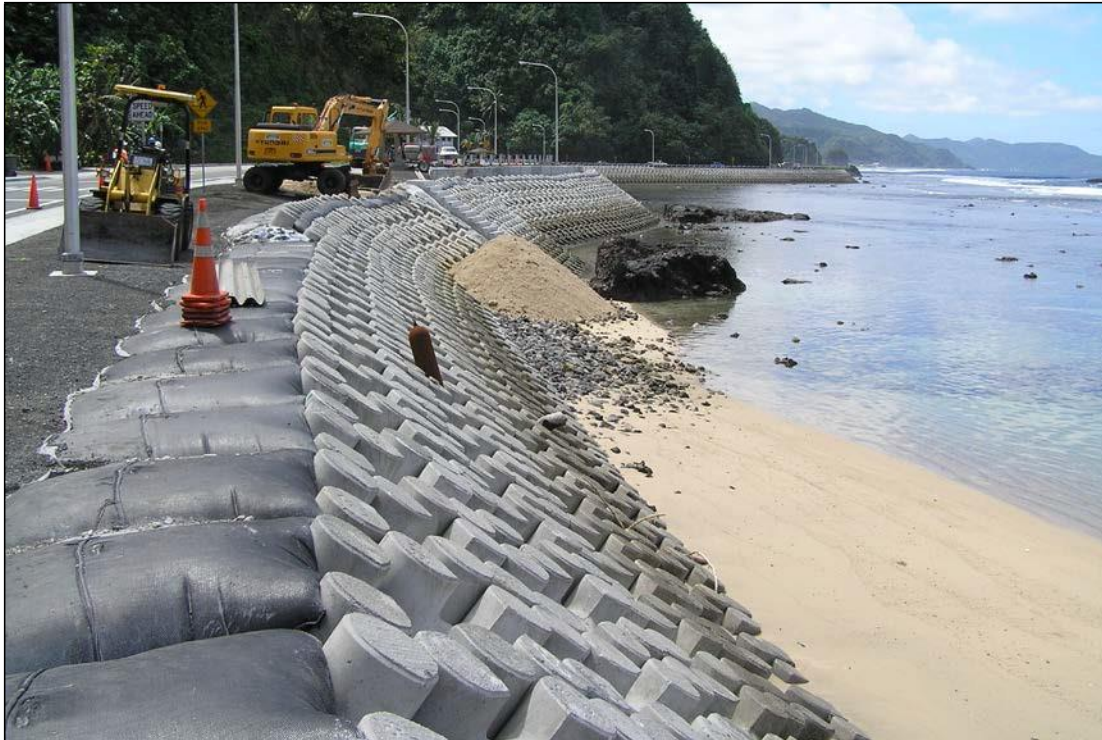
Figure A6: Tribar concrete armor unit revetment.
