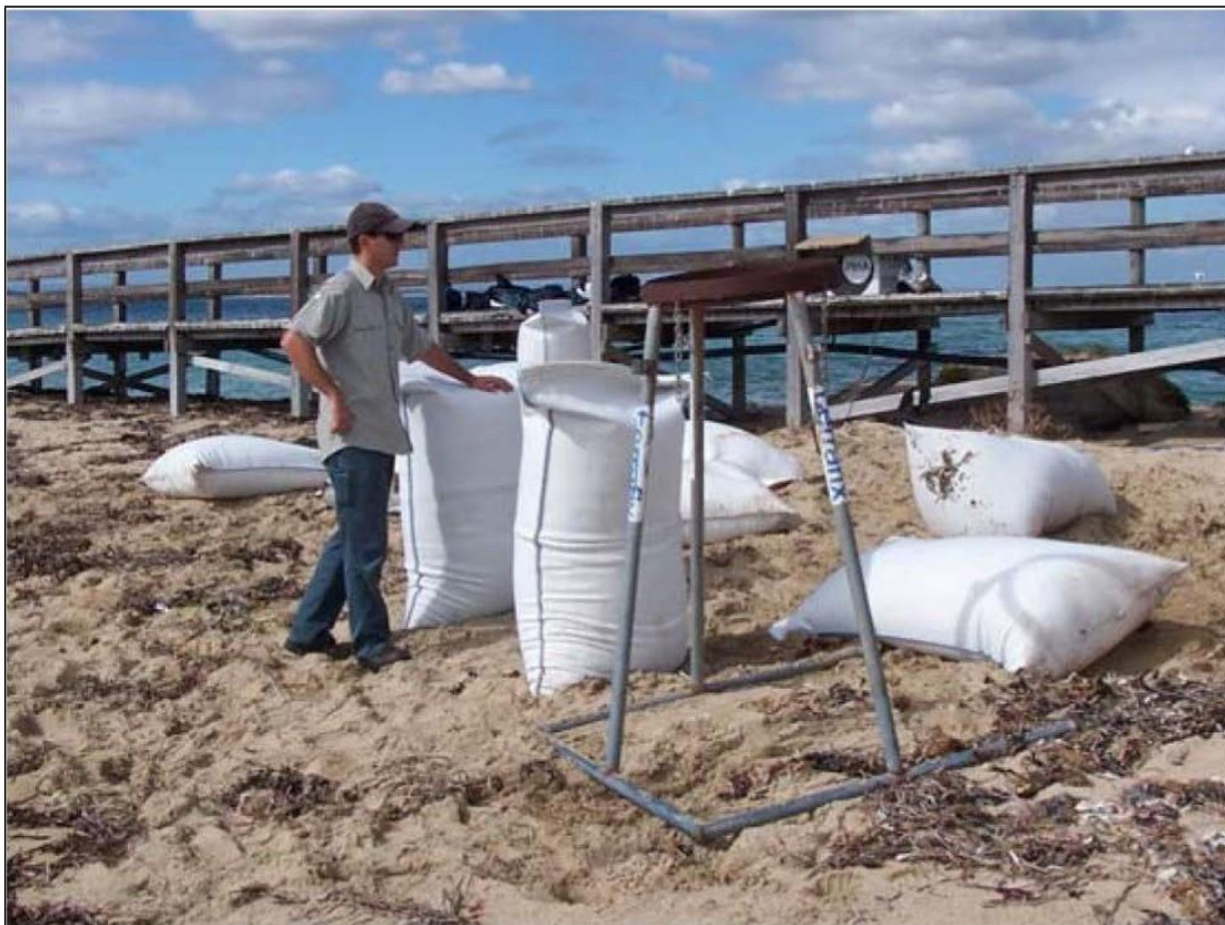
Figure A3: ELCORock Bags being filled on site.
