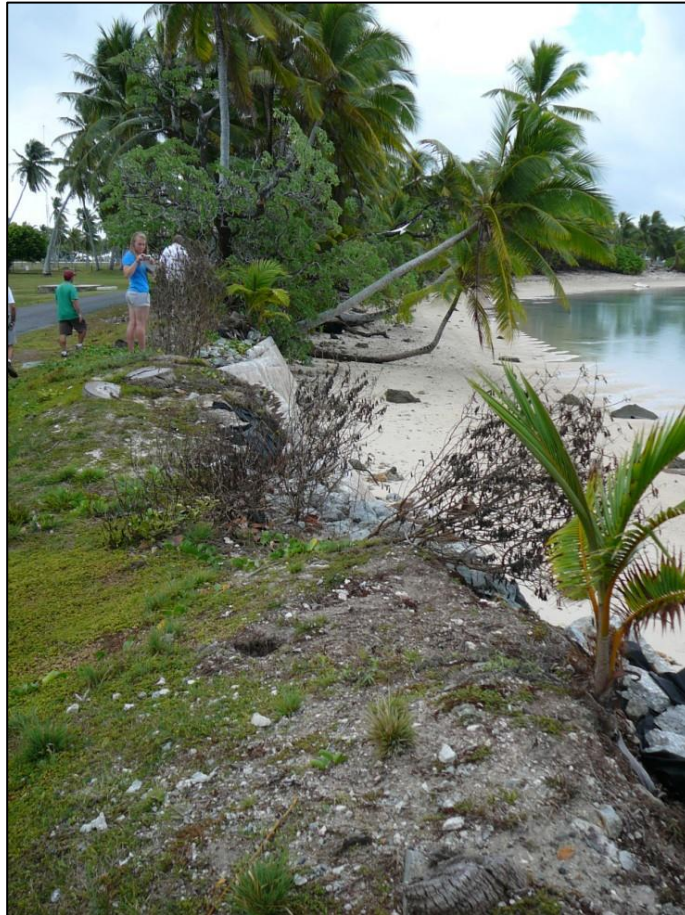
Figure 10 – Insufficient rip rap allows seawater breaching onto the road.
